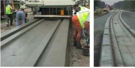
Figure 15 — Construction of Embedded Rail with paver<sup>[17]</sup> (Test-track near Best, the Netherlands. source: Strukton Railinfra)
