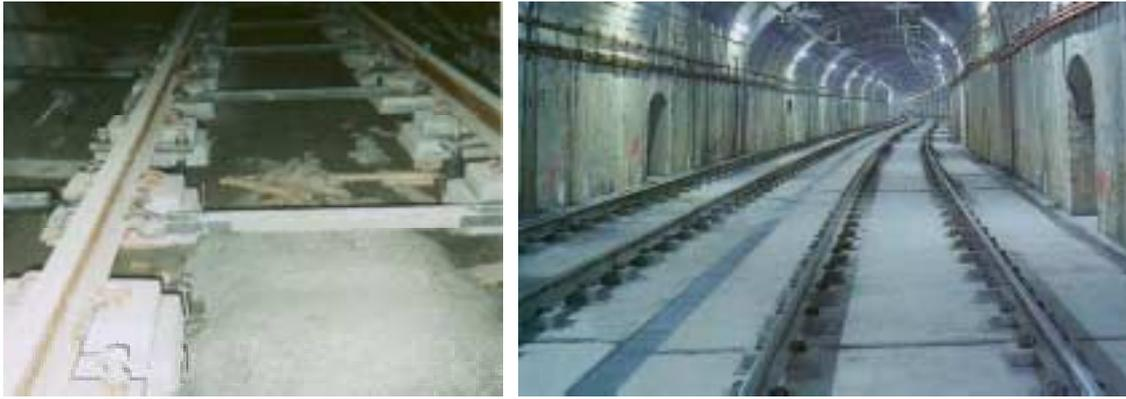
**Figure 1 Block track in construction and in use (Metro de Madrid)**
