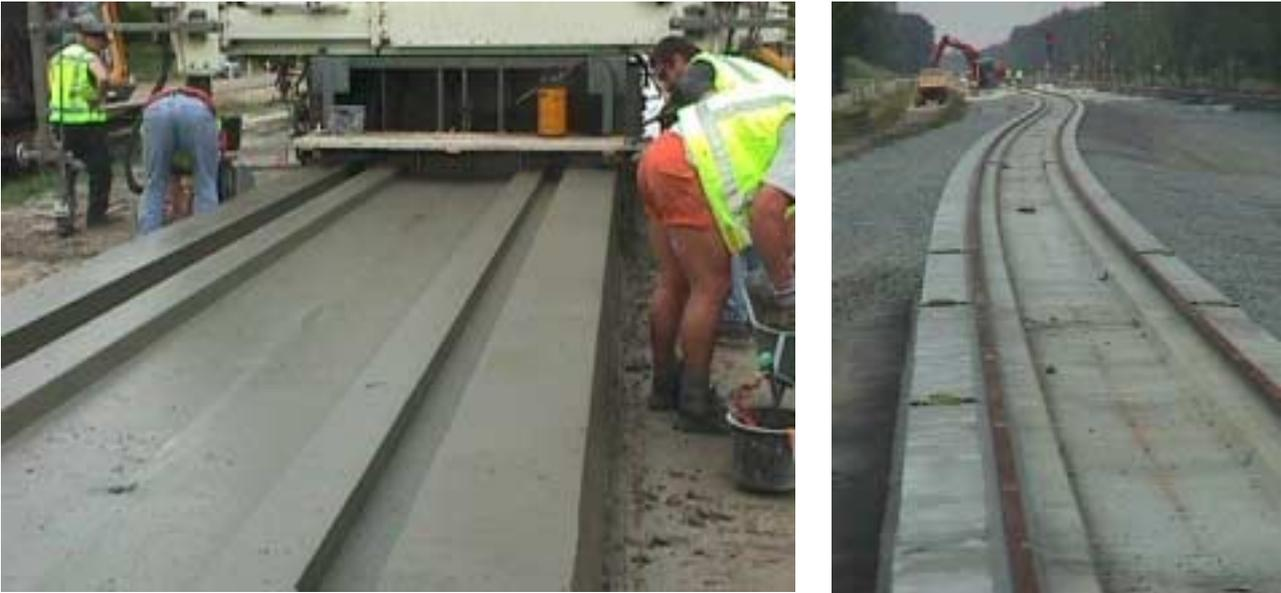
**Figure 2 Construction of Embedded Rail with paver**
